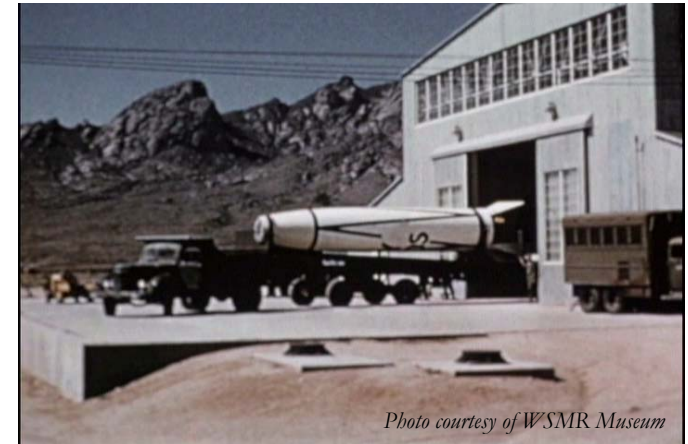
V-2 rocket #59 wheeled from building 1554 for launch on May 20, 1952.
